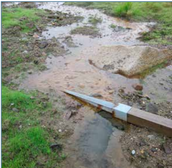
Leakage from test wells in the general area of the proposed Pebble Mine. Photo from Kendra Zamzow.
